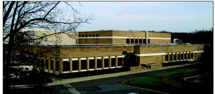
BMS CSO/DPTC facility.
