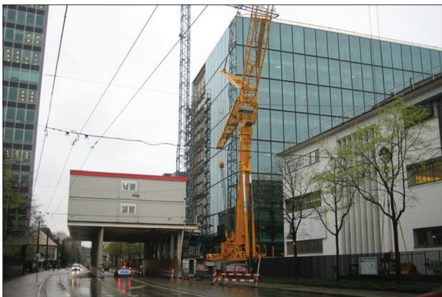
Construction staff occupied an office that was elevated above the main public roadway.
