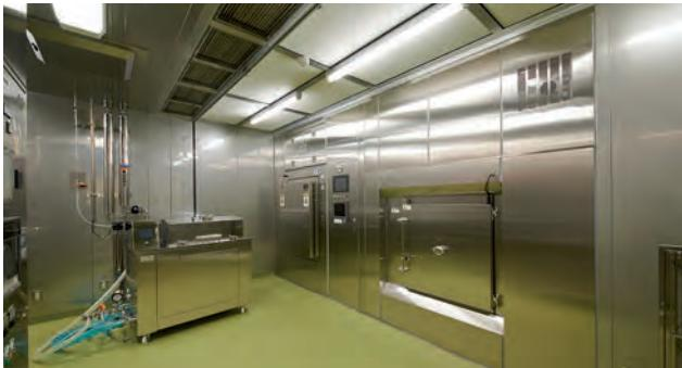
Sterilization booth, second floor—Three sterilization methods: 1) autoclave, 2) dry-heat sterilizer, and 3) dry-type VHP
