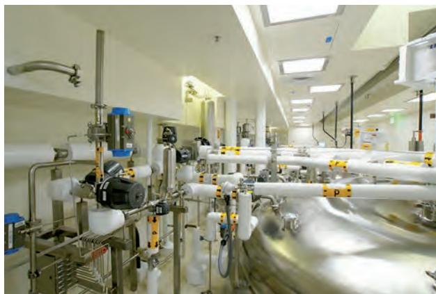
*This buffer hold area was converted from unclassified to Biozone 3.1 as part of the RTS project. The recessed area in the ceiling is an example of forethought in design, addressing the complexity in converting the area to a Biozone 3.1. This lighting system allowed for visibility and operability while working on the filter housings.*
