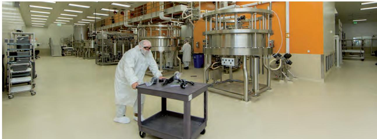
Four of the six chromatography columns in the recovery area. The LED lighting panels contribute to the over 50% reduction in lighting consumption.
