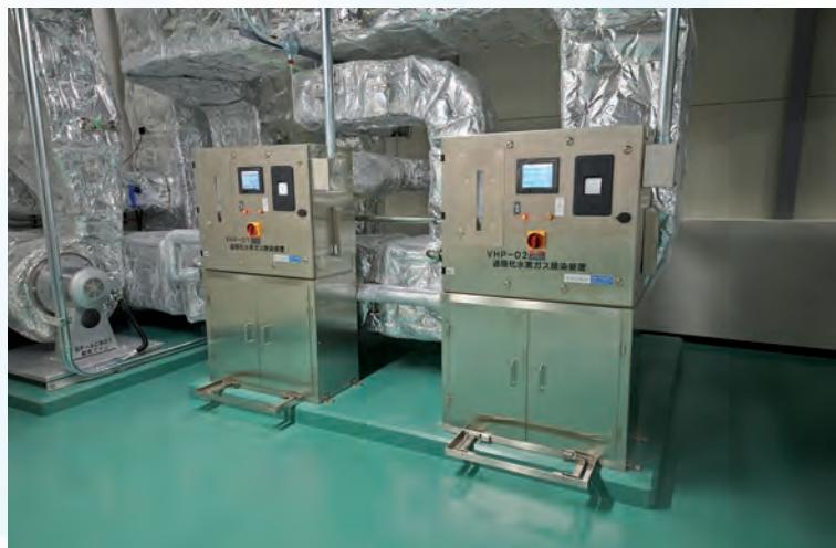
Dry type hydrogen peroxide sterilization system (in machine room, second floor)
