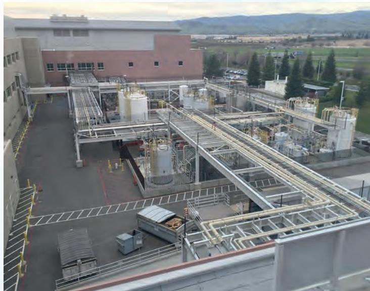
The west yard, which was expanded to supply chemicals to CCP1 and CCP2 and handle all the wastestreams from both cell culture facilities.
